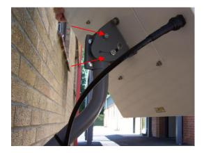
Figure 4-15 - Adjusting elevation
